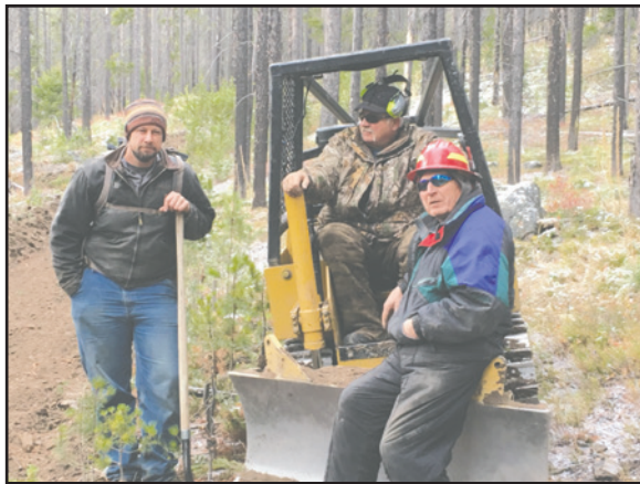
Pictured right: Josh Lattin is on the shovel, Parke Scott (Scott's Fire Service) is in the Operator's seat of the SWECO Dozer, and Harold Lear is leaning on the SWECO blade.
