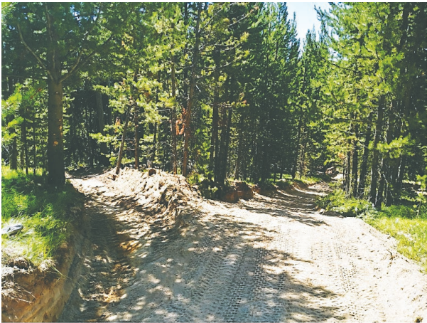
Comet Ridge Trail Maintenance Summer 2020 Water Diversion
